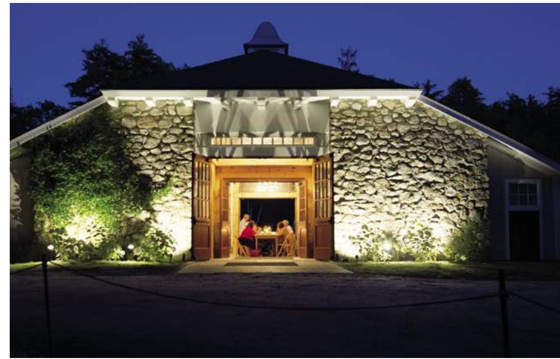
As part of the College's agritourism initiative, the Stone Barn hosted several farm-to-table dinners and dozens of community and private events this season. For more information: www.stonebarnmaine.com . Photo: Tonee Hebert.
